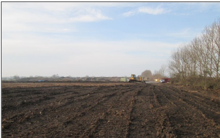
Photograph 2 – Looking from Phase 1 along the northern boundary of the site
